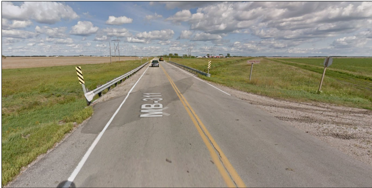
Photo 01: PR 311 bridge over Manning Canal (August 2016).
