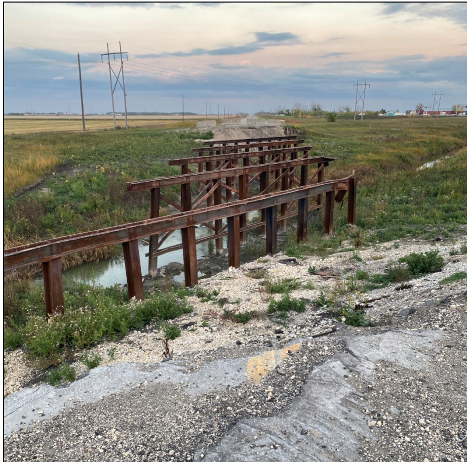
Photo 02: PR 311 bridge over Manning Canal (September 2023).
