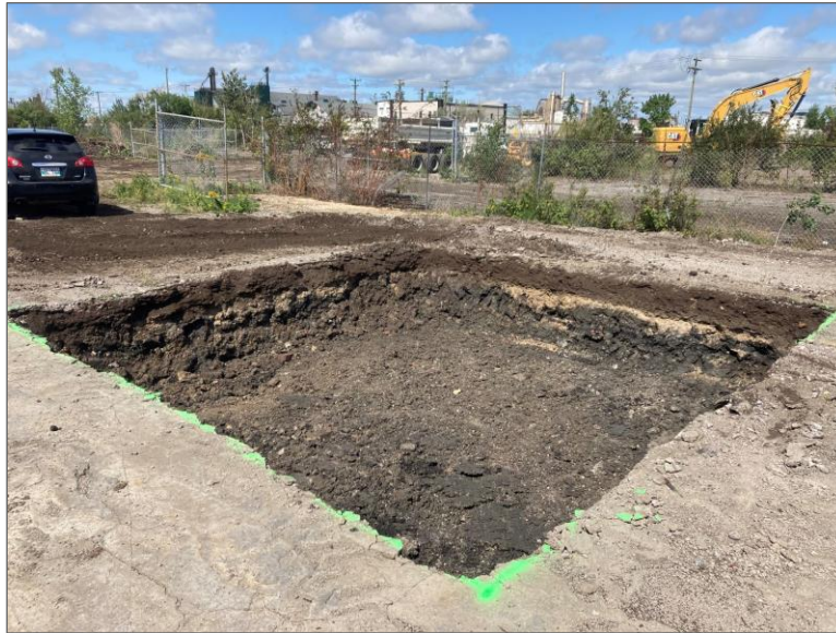
Photo 1 – Excavation 1 dimensions prior to re-excavation.
