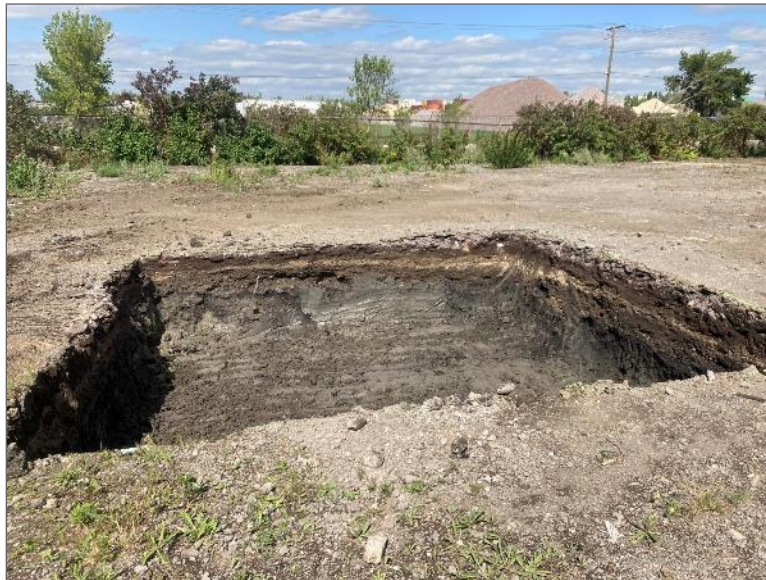
Photo 6 – Excavation 2 final limits.
