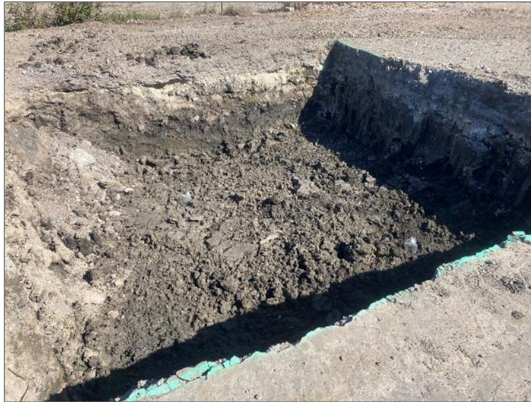
Photo 3 – Excavation 1 final limits after re-excitation.
