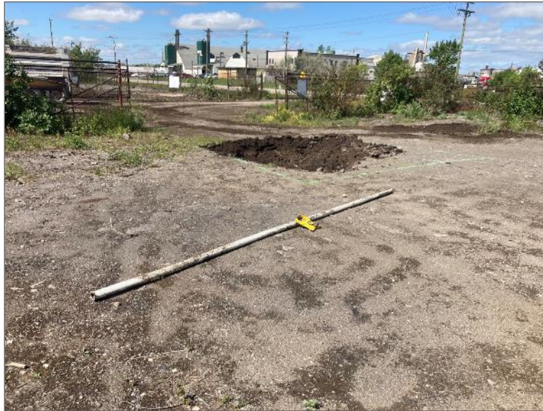
Photo 5 – PVC pipe from former monitoring well MW04 in Excavation 2.
