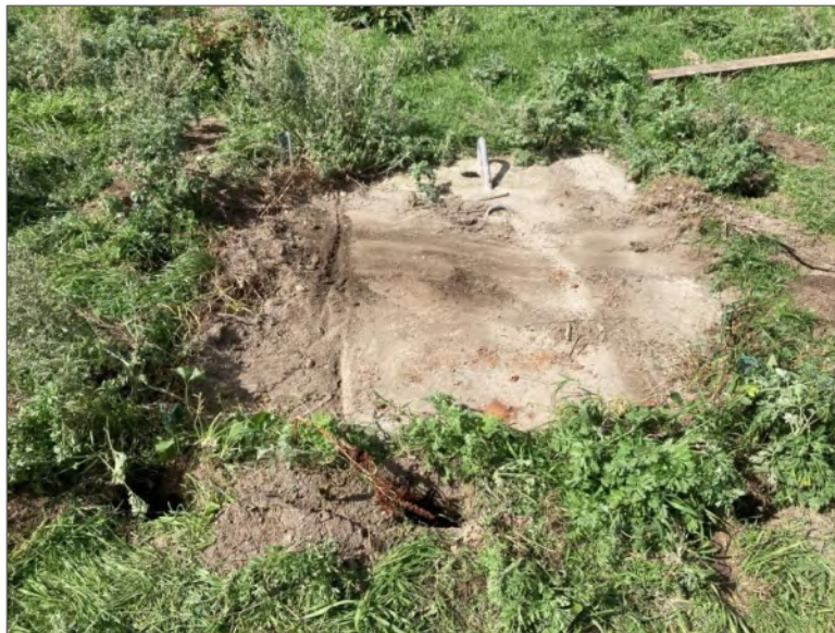
Photo 9 – Former concrete anchor exposed following removal of the hydrometric shelter.
