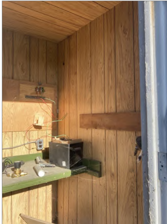
Photo 4 – Another photo of hydrometric shelter interior, showing interior ceiling and walls.
