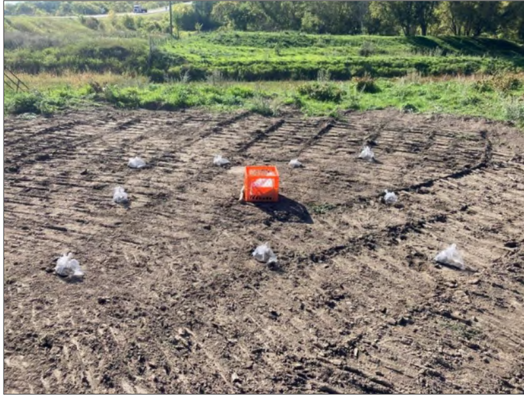
Photo 10 – Confirmatory sampling locations indicated by sample bags following soil excavation and regrading of the site.
