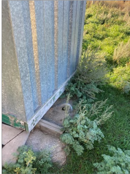
Photo 6 – Another photo of the former concrete anchor under the hydrometric shelter.
