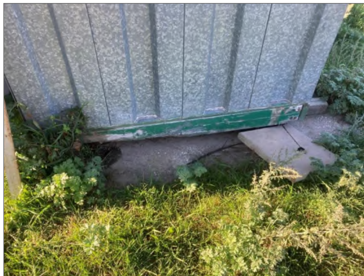
Photo 5 – A former concrete anchor under the hydrometric shelter.
