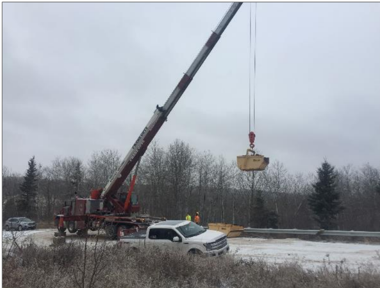
Photo 2 – Metal bin used for recovering excavated soil material from the excavation area.
