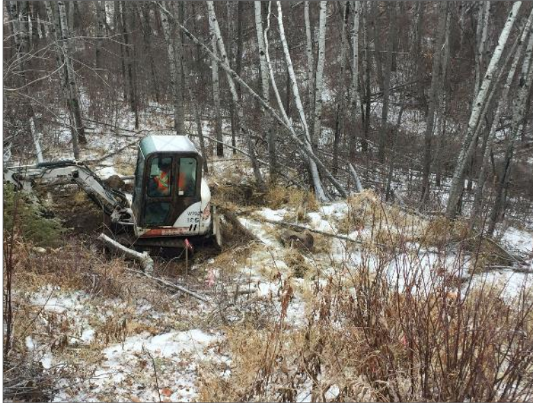
Photo 1 – Excavation activities at the roll over incident area at the Site.
