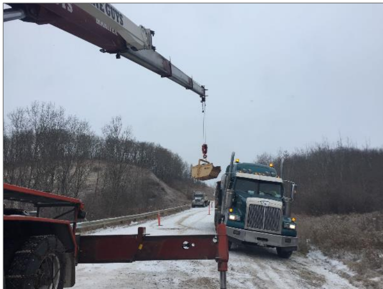
Photo 4 – Excavated soil material being loaded for off-Site transport.
