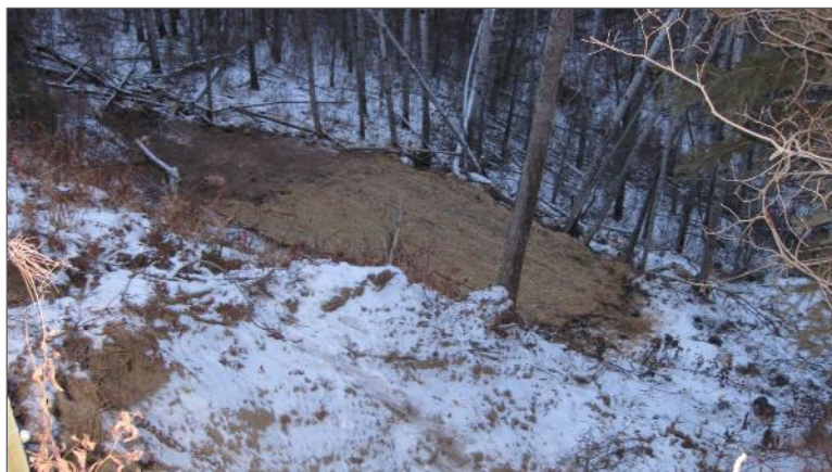
Photo 11 – Final appearance of the backfilled excavation.
