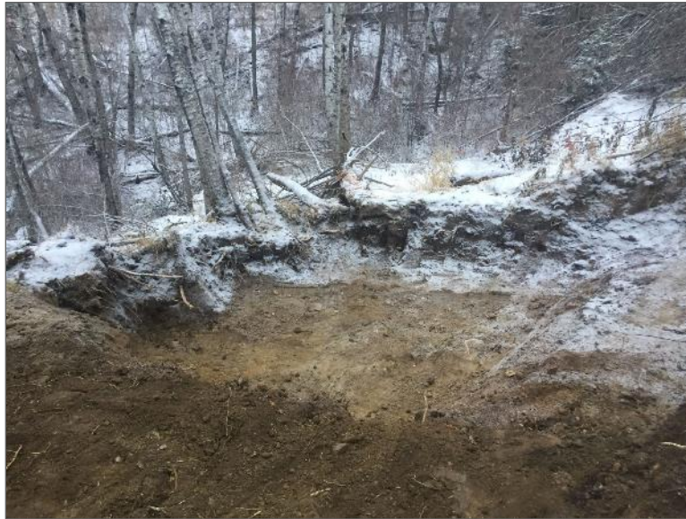
Photo 5 – Final limits of the excavation. Photo taken facing north.
