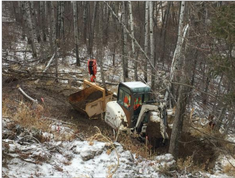
Photo 3 – Excavation activities at the Site.
