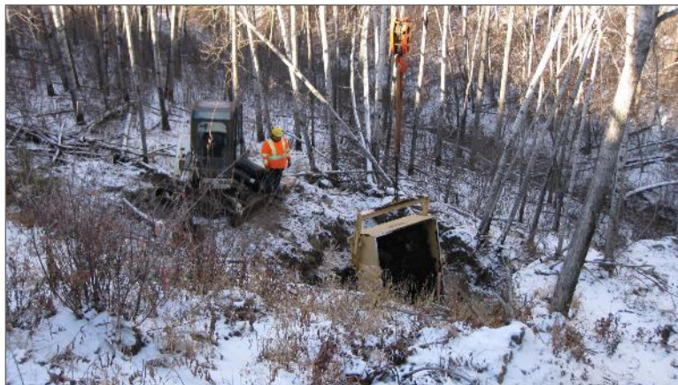
Photo 8 – Backfilling activities at the Site.
