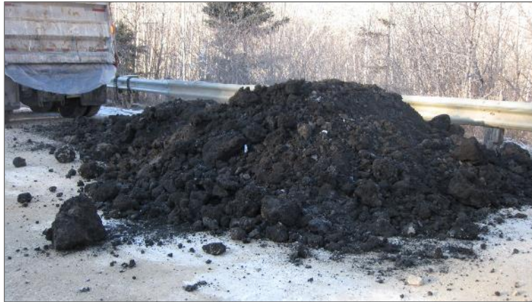
Photo 7 – Topsoil backfill material used for backfilling the excavation.
