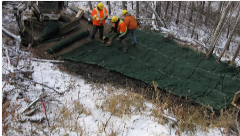
Photo 9 – Installation of the PYRAMAT® 25 turf reinforcement mat post-backfilling of the excavation.
