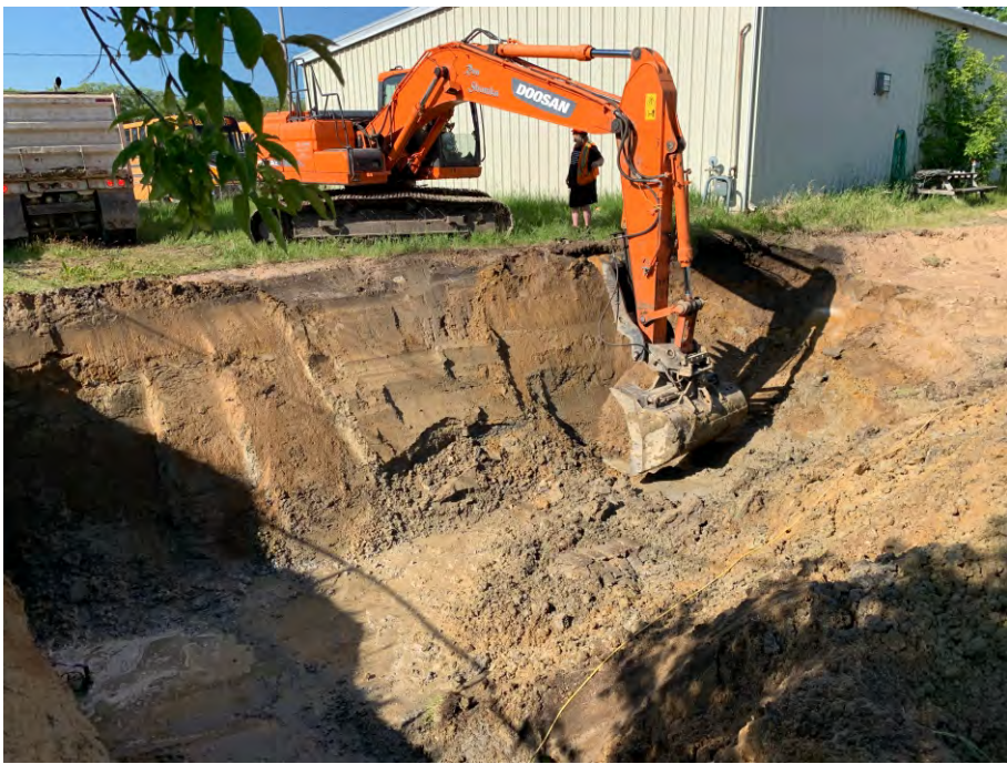
Photo # 1: View of excavation near bus garage - June 2021.
