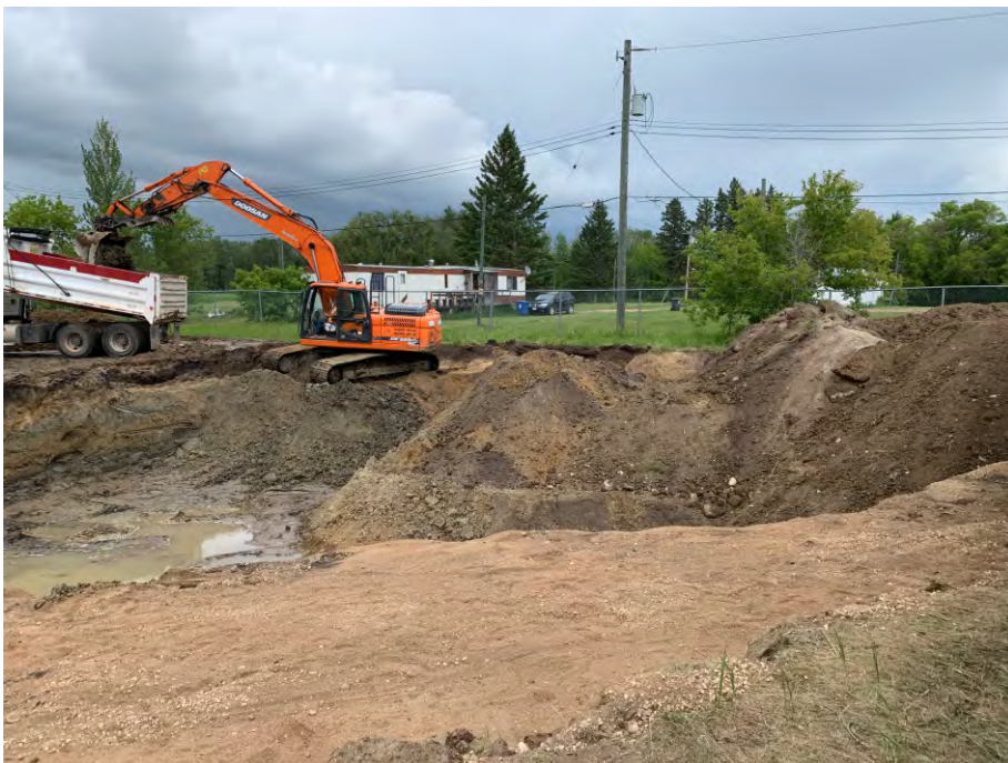
Photo # 4: Final excavation edge on right, backfill on left - June 2021.
