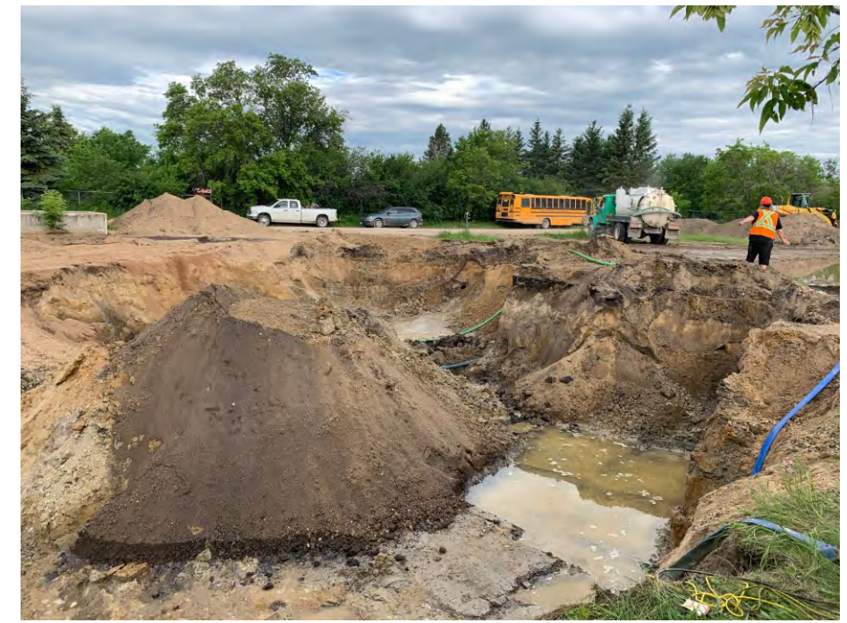
Photo # 3: Preparing to remove collected groundwater - June 2021.
