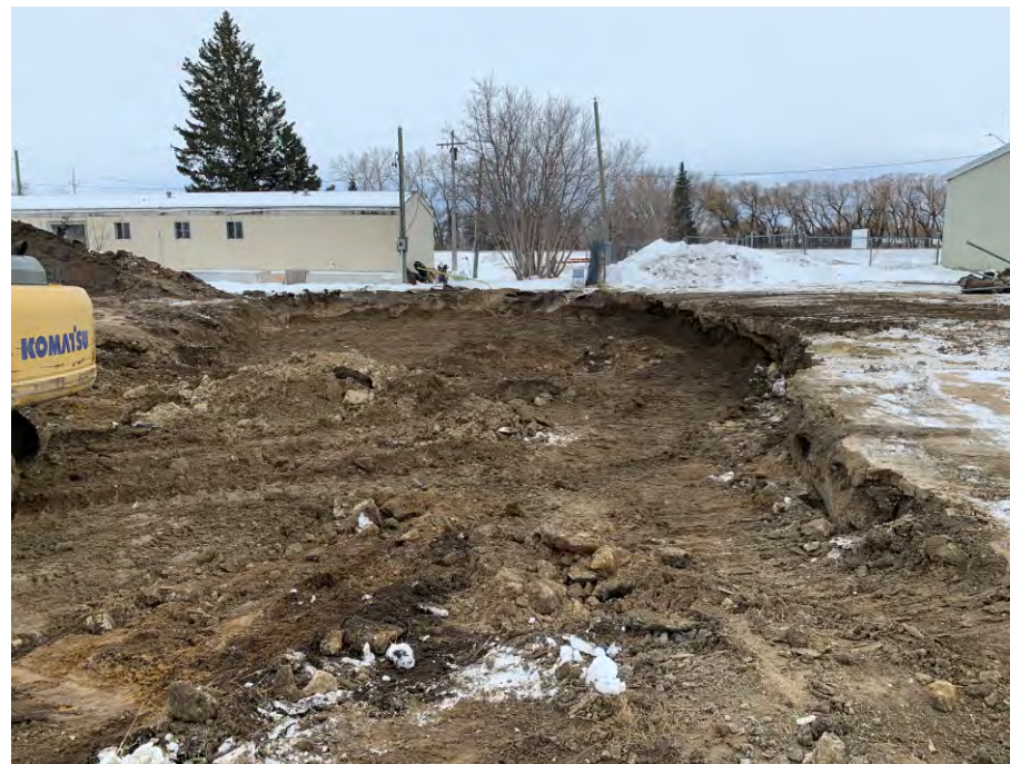
Photo # 6: Backfilling of excavation - November 2021.
