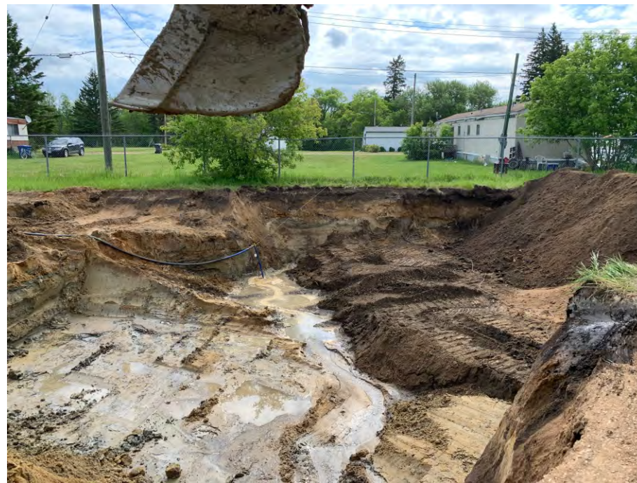
Photo # 2: Excavating near concrete dyke - June 2021.
