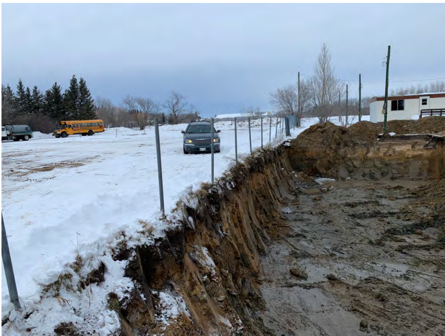
Photo # 4: Excavation prior to advance into bus garage property - November 2021.
