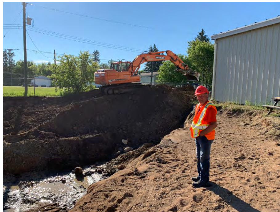
Photo # 5: Backfilling of excavation - June 2021.
