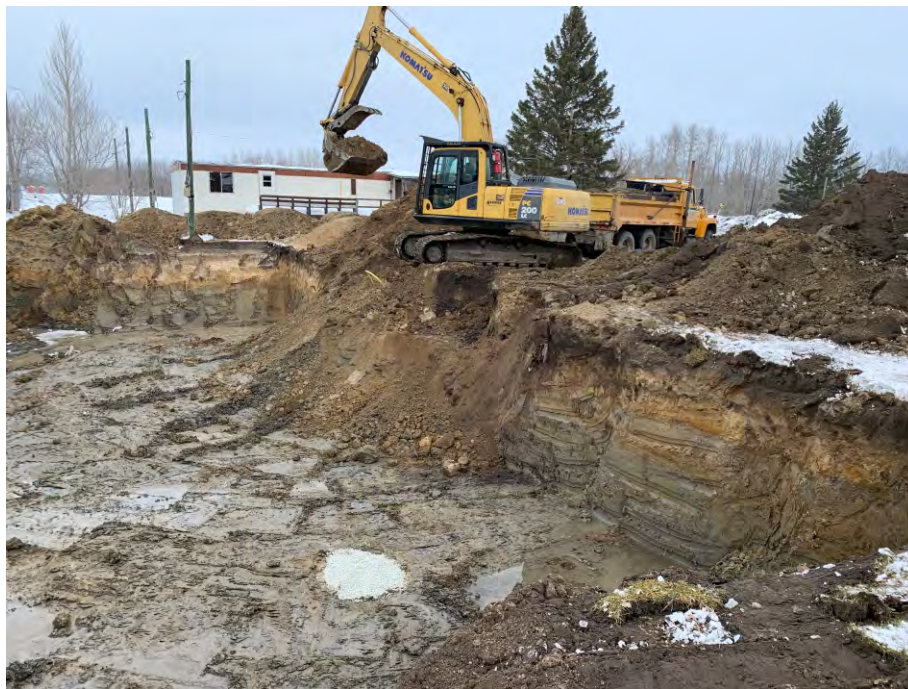
Photo # 2: Excavating on adjacent property facing north - November 2021.
