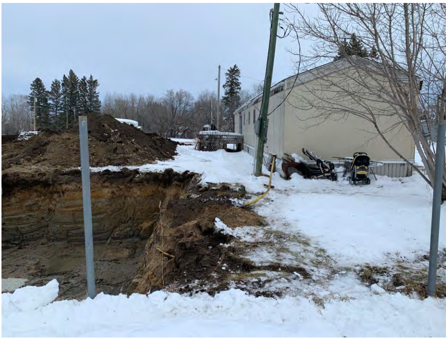
Photo # 1: View of excavation, adjacent property - November 2021.
