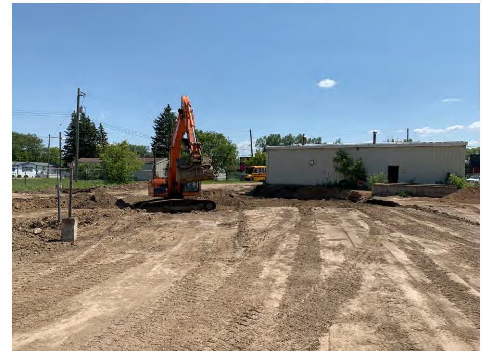
Photo # 6: Backfilling of excavation - June 2021.
