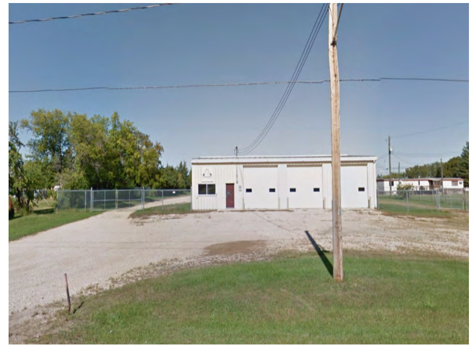
Photo # 6: Front view of Bus Garage, residential buildings at right background.
