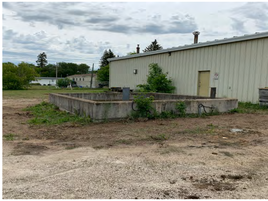
Photo # 2: View of remaining concrete petroleum storage tank containment dike.
