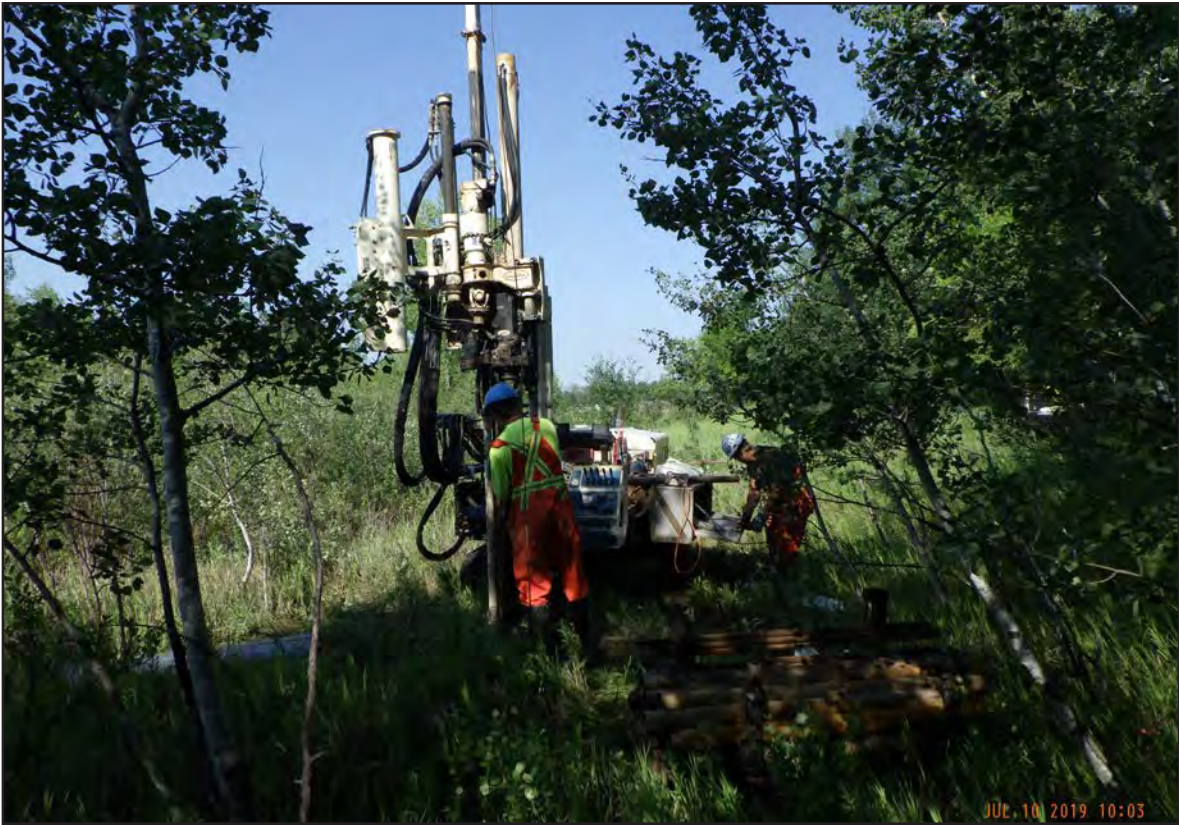
View looking west of monitoring well MW13 being advanced to the north of the IWWTF.
