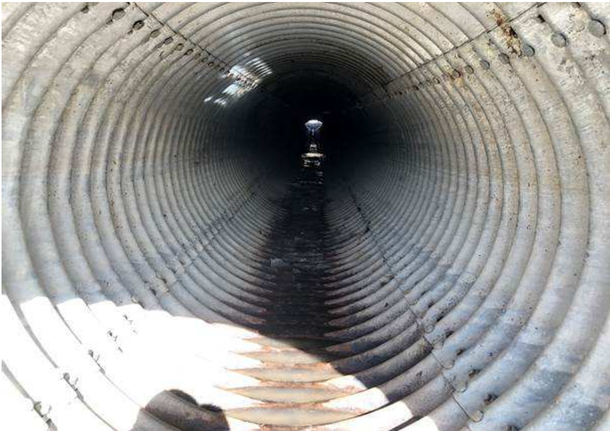
Photo 20: April 13, 2019 view looking north from the south end of the east culvert. Standing water is present in the middle of the culvert; no product or hydrocarbon sheen observed in surface water.
