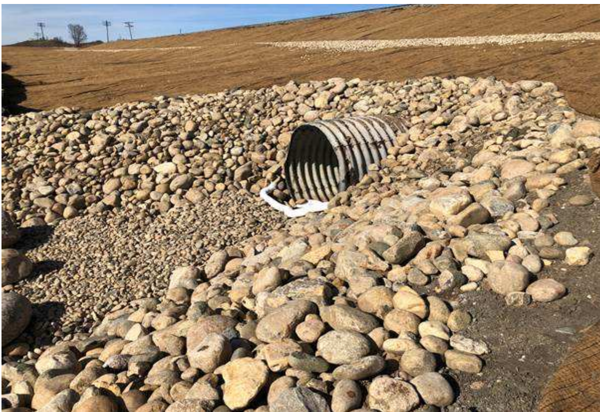
Photo 21: View of south end of east culvert after absorbent boom deployment – no outflow of surface water.
