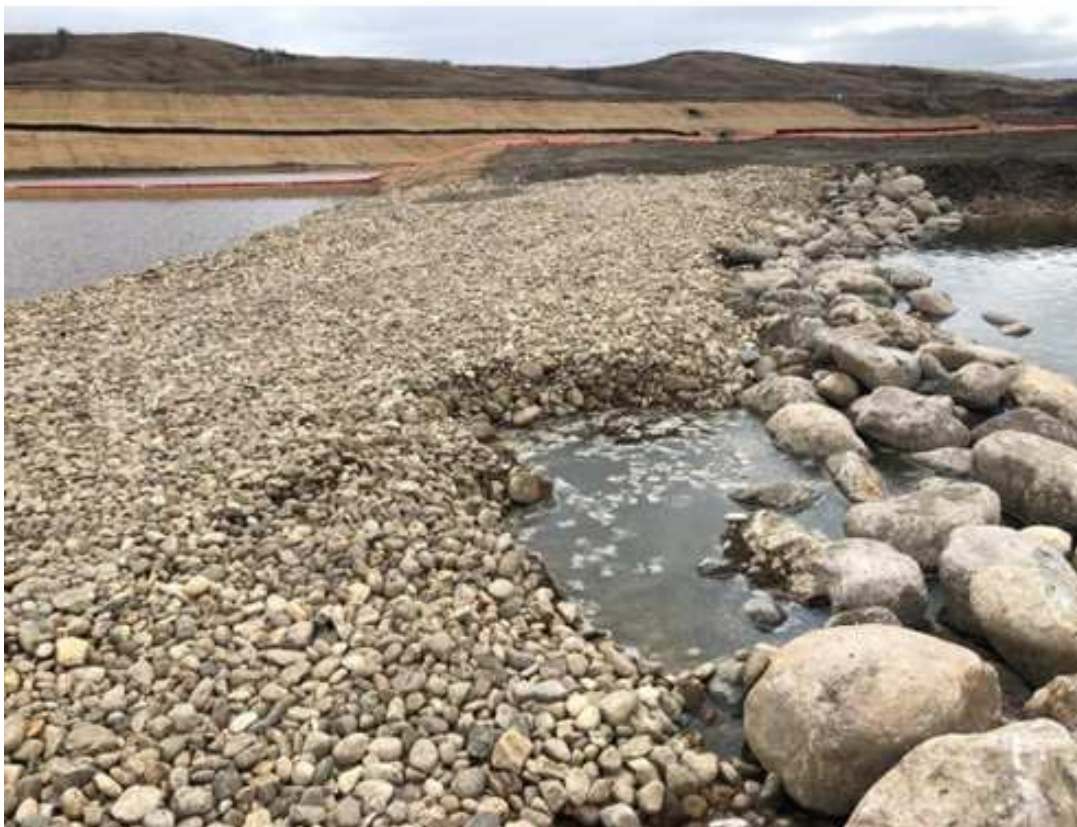
Photo 16: Area of subsidence within the south berm.
