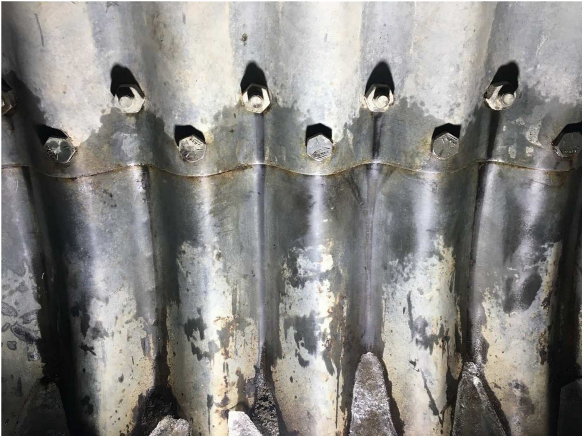
Photo 25 – Seepage in east culvert after cleaning as observed on April 14, 2019.
