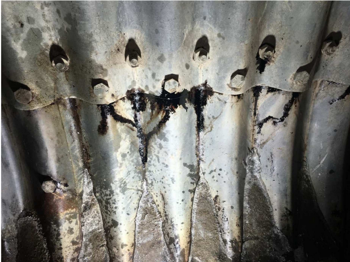
Photo 24 – Seepage in east culvert prior to cleaning as observed on April 14, 2019.
