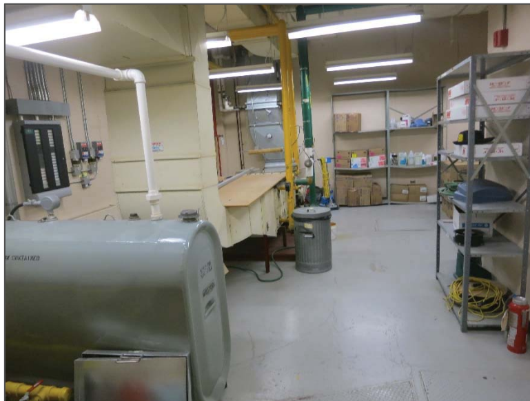
Photo 6 – First floor mechanical room (location of decommissioned UST) and diesel AST on the left.
