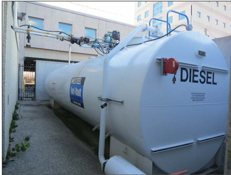
Photo 5 – 35,000 L AST on the exterior portion of the Site.
