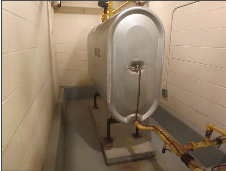
Photo 7 – View of diesel AST (one of two) in a room off the third floor generator room.
