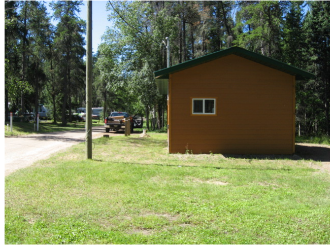
Photo 2. South view of pumphouse and well field.
