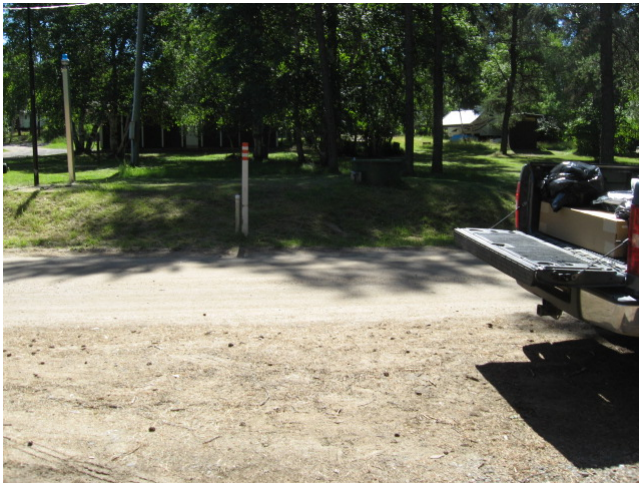
Photo 9. East view of monitoring well MW-1 and sewage lift station.
