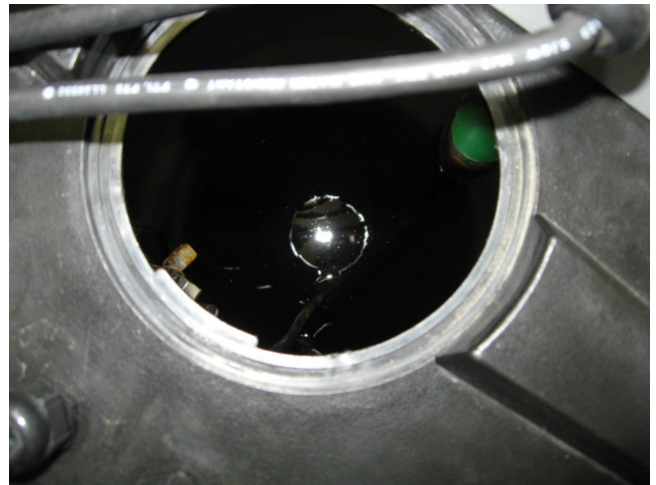
Photo 16. Water in storage tank with dark staining on sides of tank.
