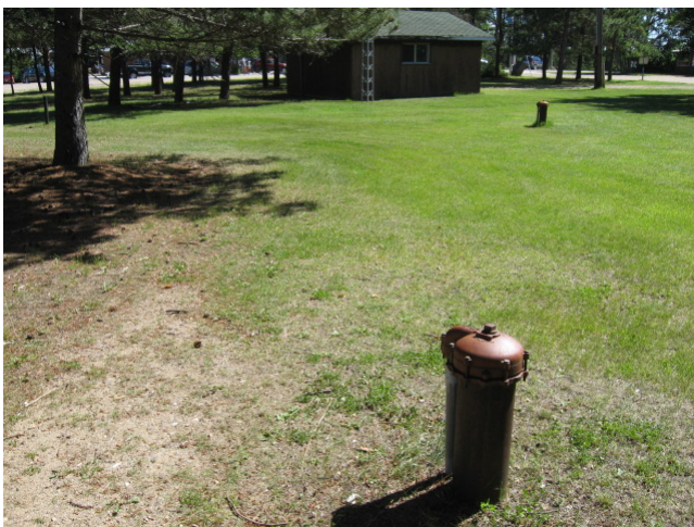
Photo 5. North-east view of former pumphouse and well field.
