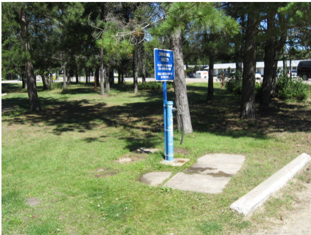
Photo 9. Community drinking water tap next to the former pumphouse.
