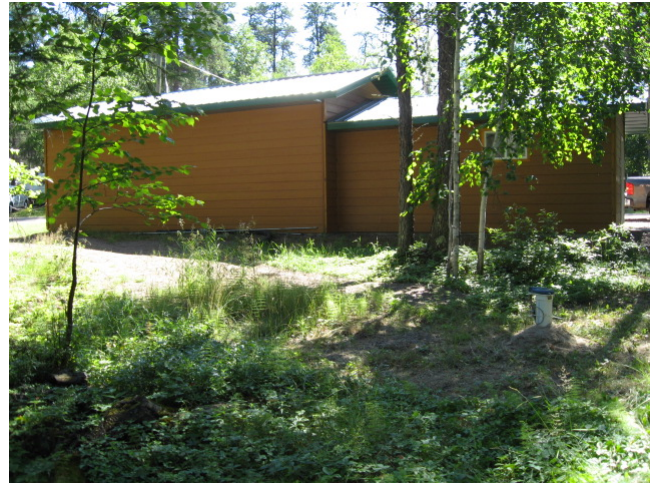
Photo 4. East view of supply well PW-5 and pumphouse.
