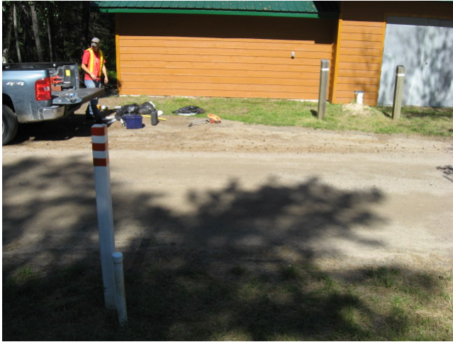
Photo 1. West view of the current pumphouse and supply well PW-1A.
