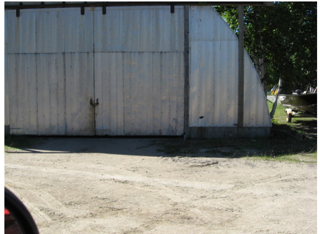
Photo 16. South view of workshop 2.
