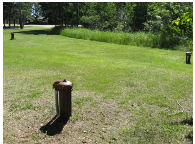
Photo 6. East view of former supply wells Well 1, Well 2, and Well 3.
