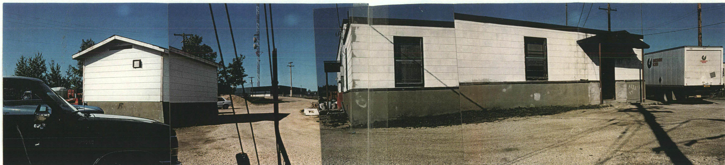
Photo 3 View of the Cranberry Portage Diesel Site looking West
