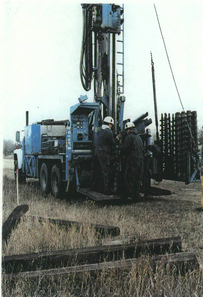
Photo 5 Paddock Drilling's Canterra Drill (Photo from another Project)
