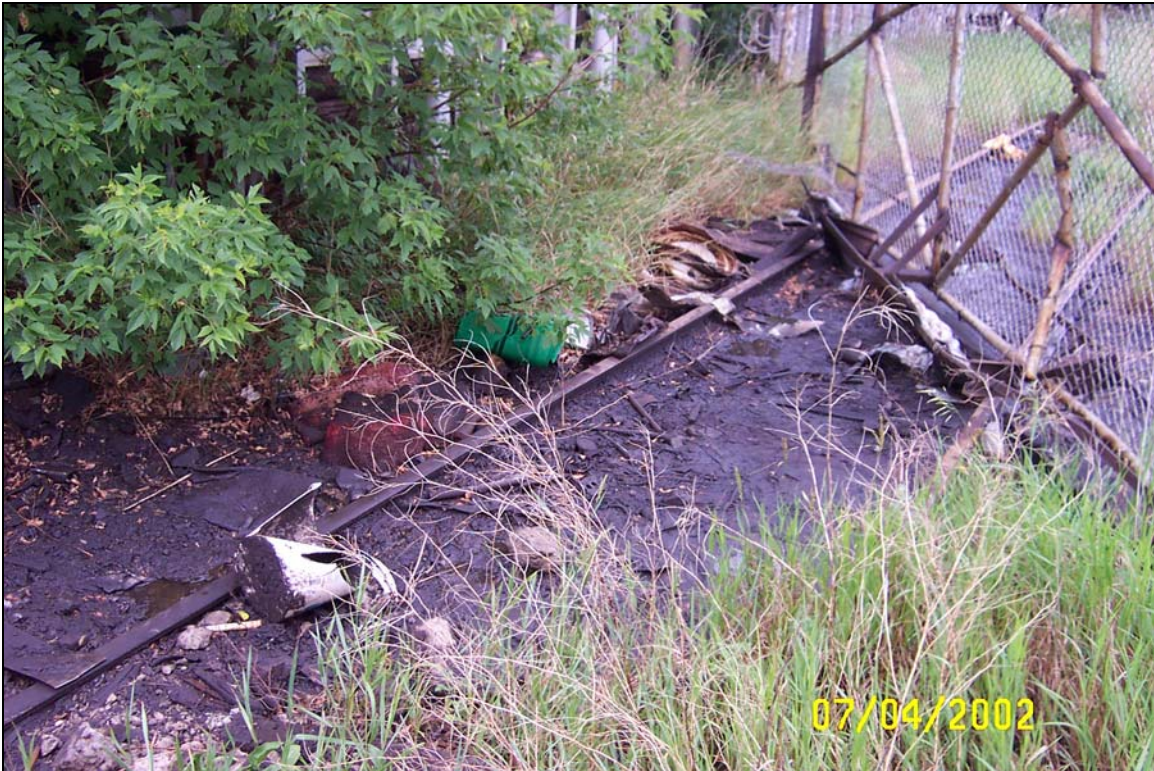
Photograph 22: Area of extensive staining located on the abandon spur line along the southern edge of the property at 9 First Street.
