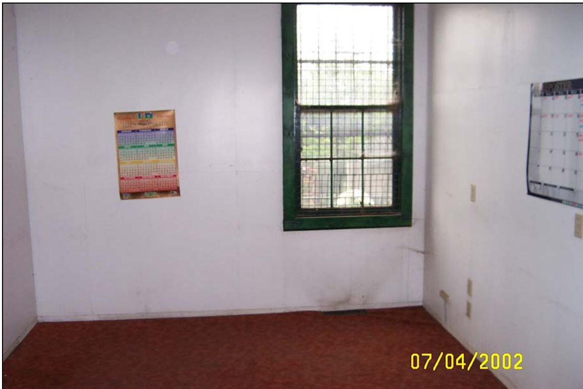
Photograph 8: Typical office room located within the build located at 9 First Street.
