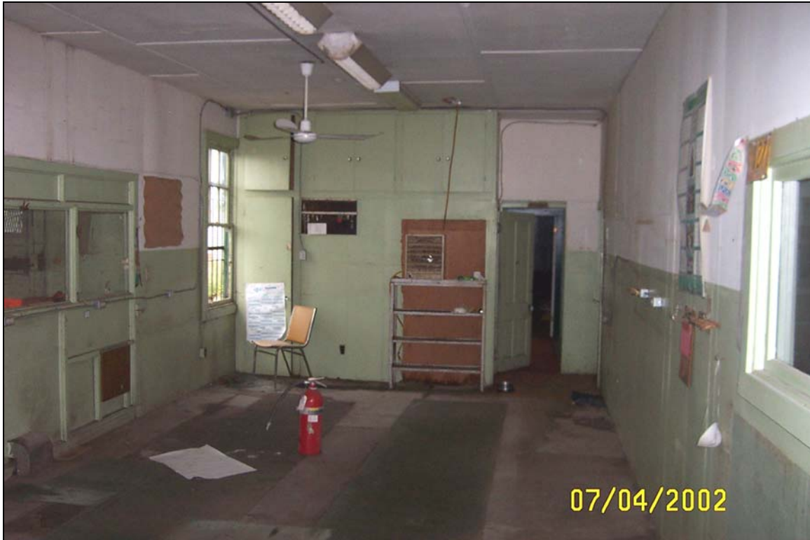
Photograph 7: Typical office area located in the northwest corner of the building at 9 First Street.
