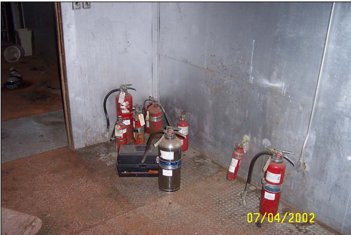
Photograph 10: At least nine (9) fire extinguishers are located in a room between the office area and the shipping area.
