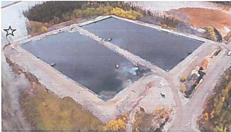
Figure 2 Aerial View of Copper Ponds looking Northeast
