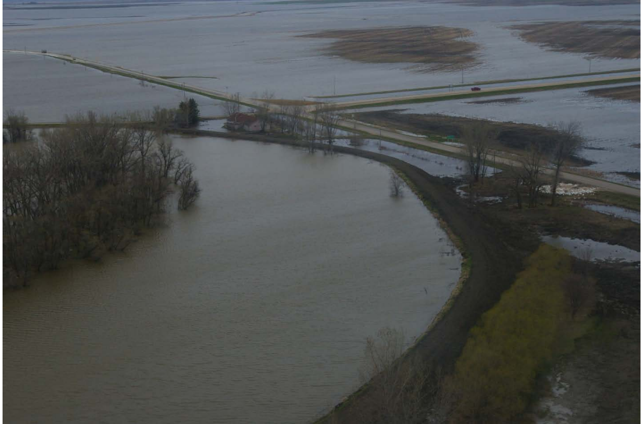
Figure 28: Photograph of the Assiniboine River and dikes in the vicinity of Baie St. Paul, taken on May 15, 2011. Note that there is freeboard remaining on the dikes (they are not in danger of being overtopped).
