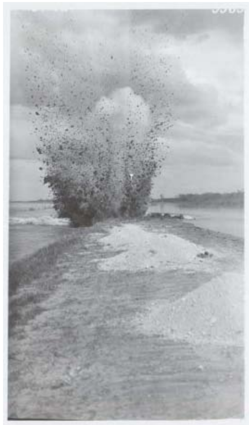
Figure 15: Photograph from 1922 showing blasting of the Winnipeg-Portage highway to allow flood waters to pass without destroying the entire length of road (Attwood, 1923).
