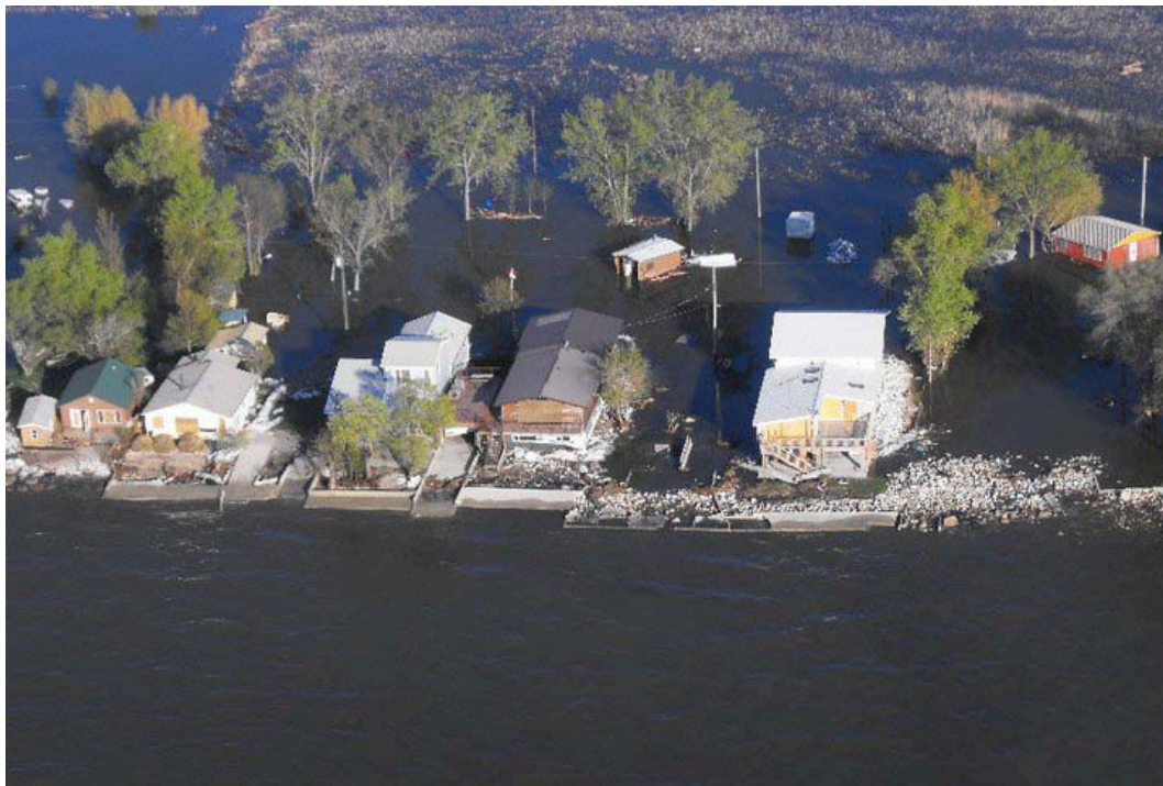
Figure 51: Photograph illustrating damage to cottages in the Twin Lakes Beach area, on the southern shores of Lake Manitoba.
