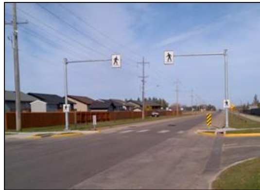
Overhead-Mounted Signed Crosswalk
