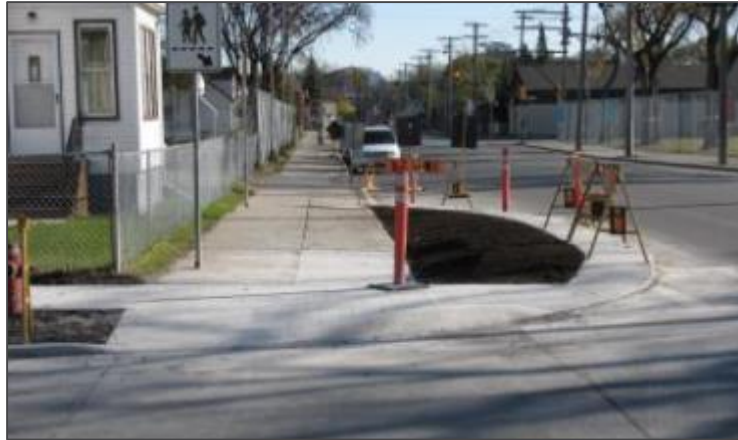
Curb extension under construction near a school in Winnipeg. 9
