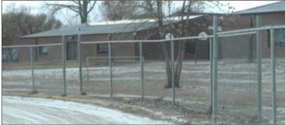
Chain-link fence limits access to school bus loading area.
