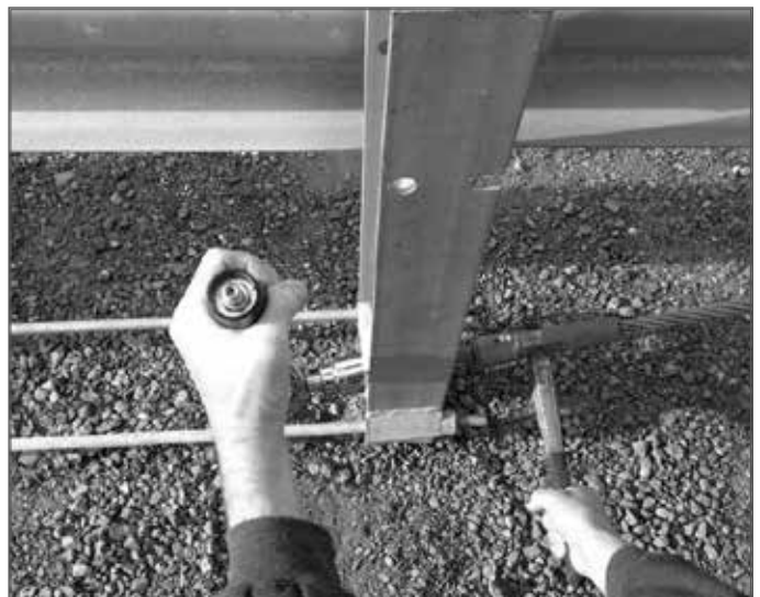
Torque cable nut to 60 ft.-lb. at Post 2
