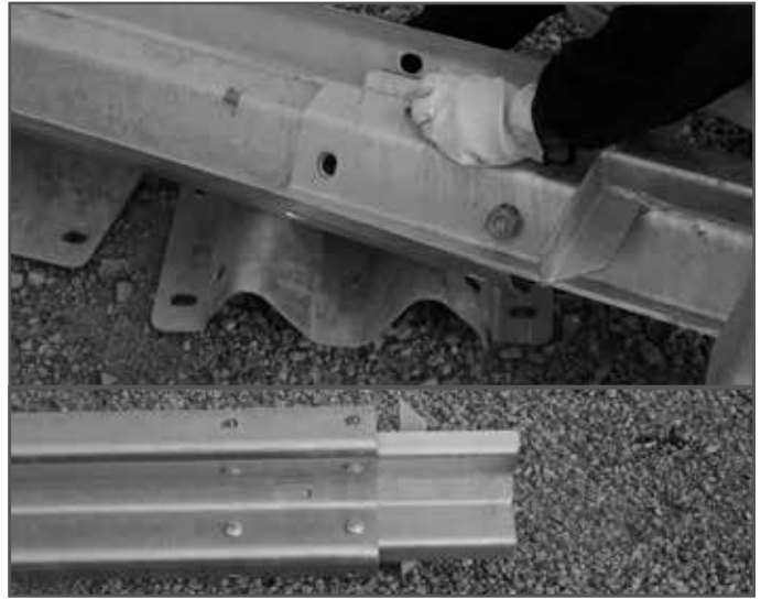
Attach Slider Bracket to Rail 2.
