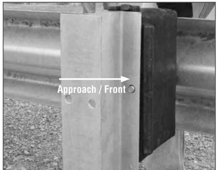
Attach Rails to Posts
