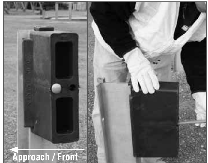
Install Blockouts
