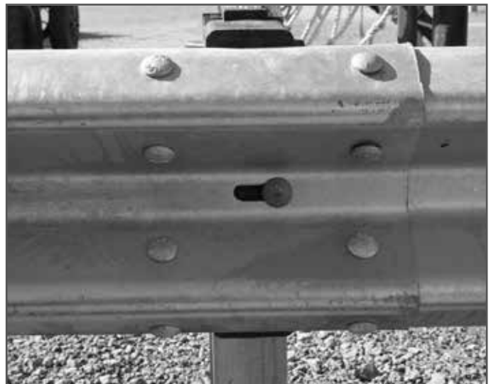
Standard Bolts at Rail 3 and 4 Connection
