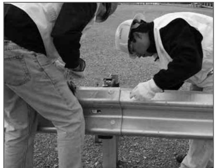
Shear Bolts at Rail 2 and 3 Connection
