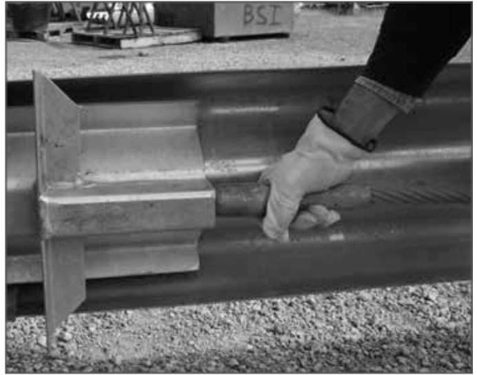
Install Trailing / Back End of Cable Through Bracket at Post 3
