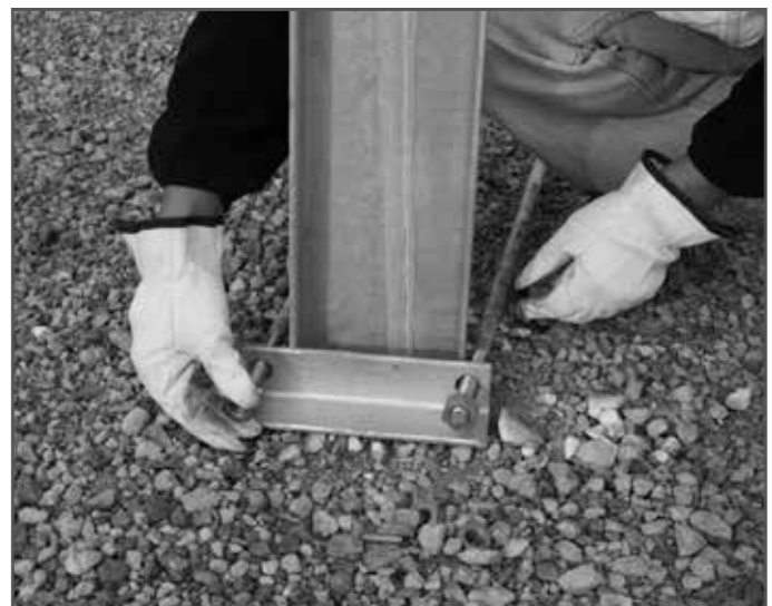
Ground Strut Tension Rods Attached at Post 1
