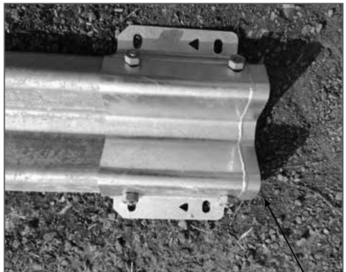
Attach Slider Panel (Front) to Rail 1.
