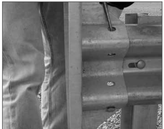
Install Impact Head at the End of Rail 1
