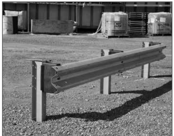
Existing Trailing / Back Guardrail
