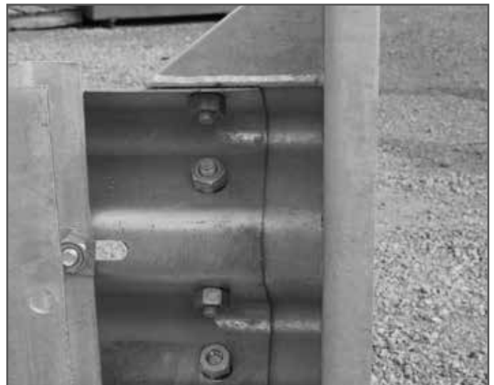
Impact Head Installed
