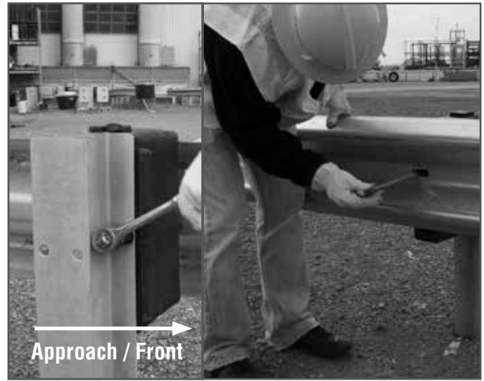
Attach Rail 2 at Post 4
