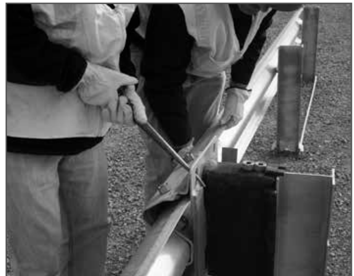
Connect Rails 1 and 2 at Slider Assembly
