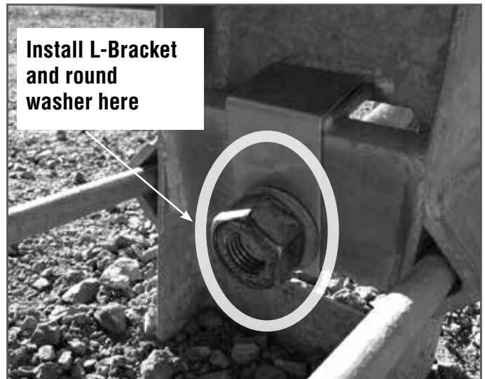
L-Bracket installed at Post 2 Prior to Tightening
