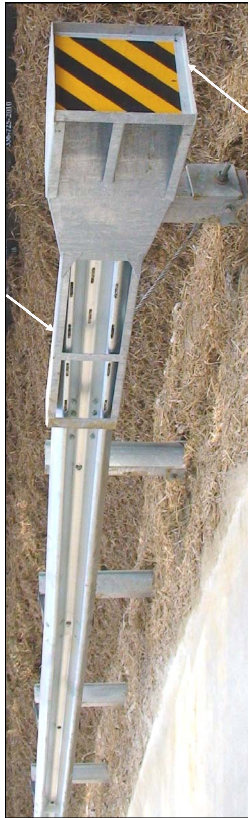
Impact Head Feeder Guide Chute
