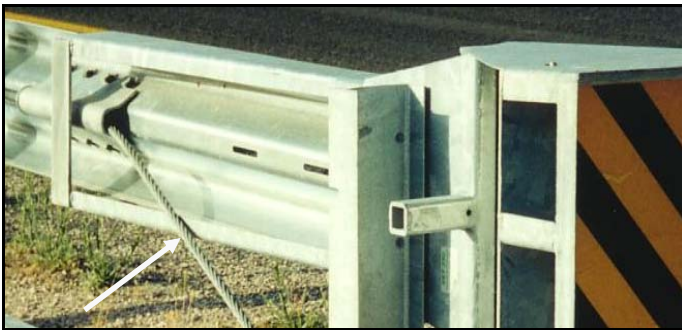
The SKT-SP cable is fed inside through the feeder chute. The SKT feeder chute is longer than the FLEAT
