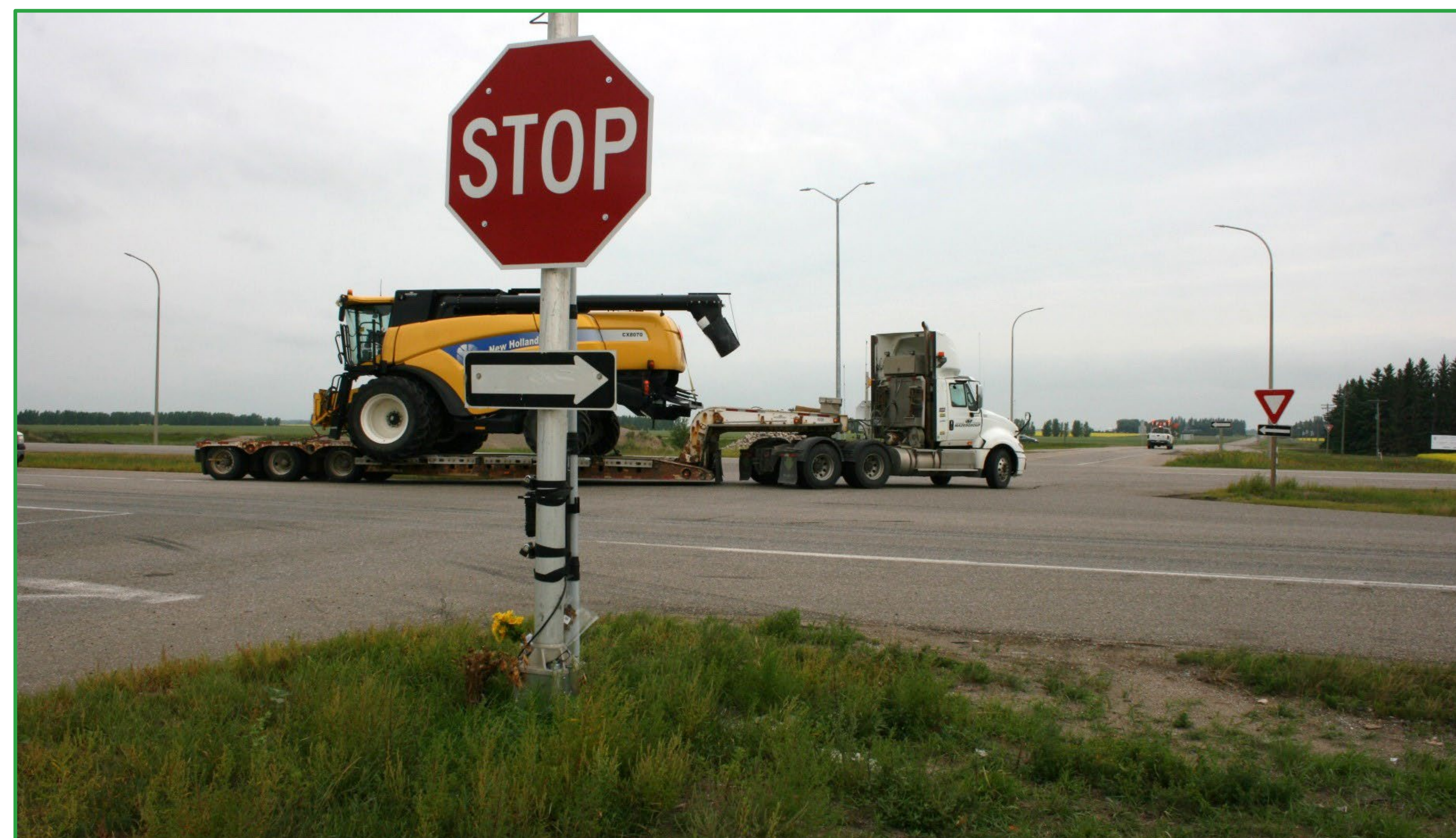
PTH 1 and PTH 5 intersection looking north.
