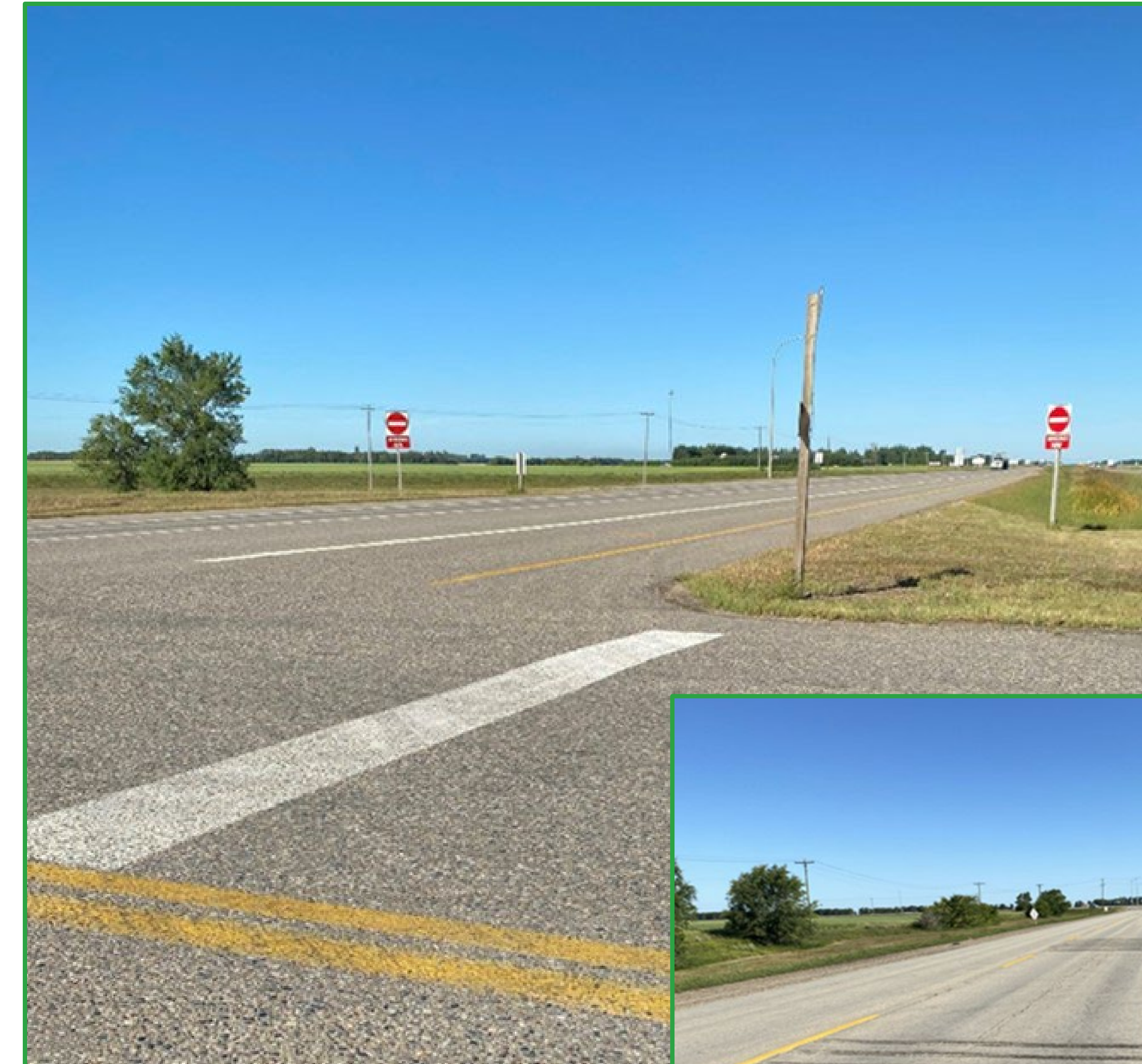
Refurbished pavement markings at the intersection.
