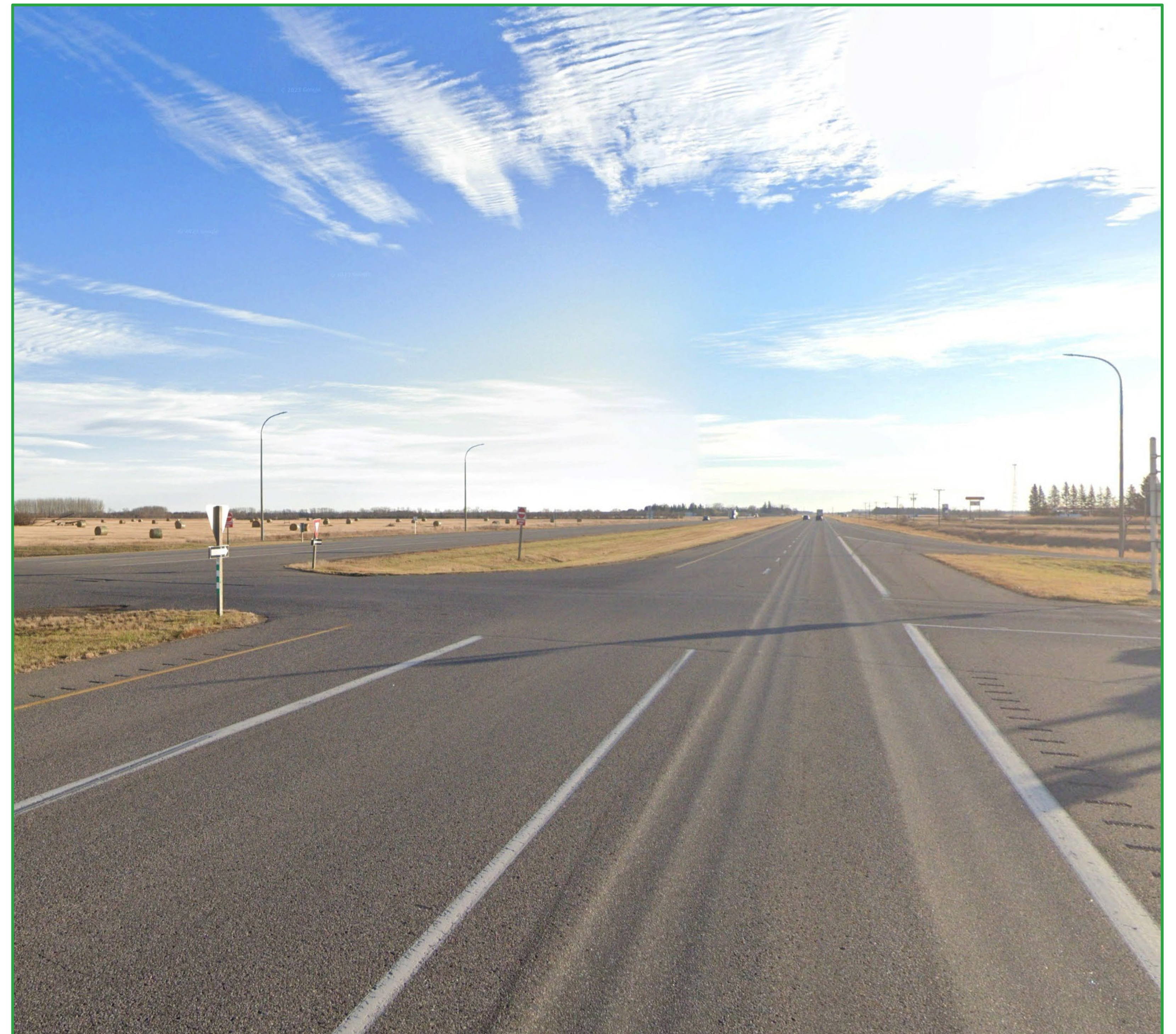
PTH 1 and PTH 5 intersection looking east.
