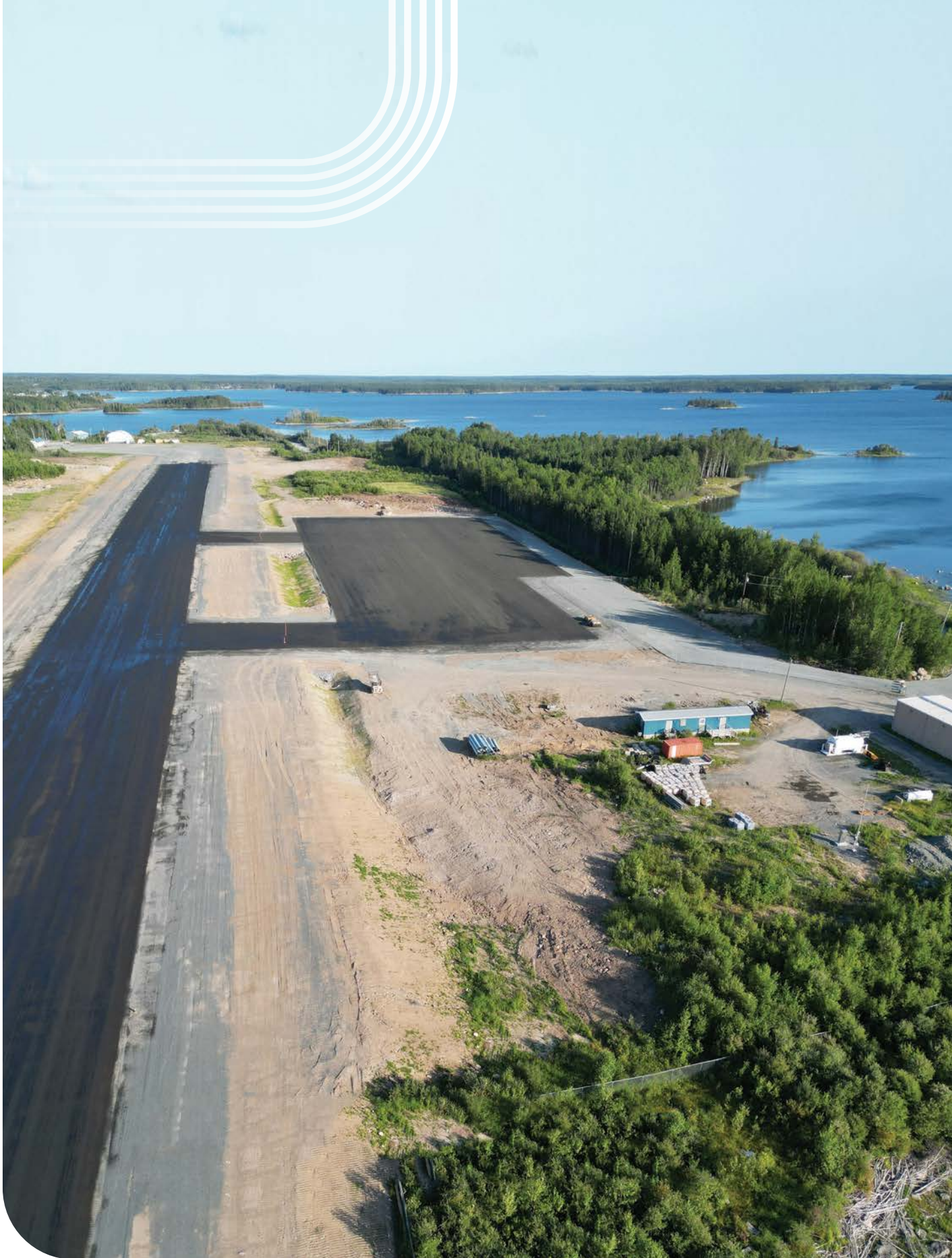
God's Lake Narrows Airport airside rehabilitation project
