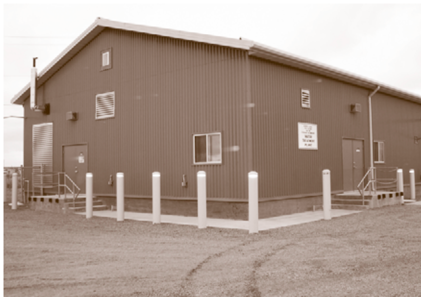
Assets like the Brochet-Barren Lands water treatment plant are expensive to operate and maintain, but essential to community health.
