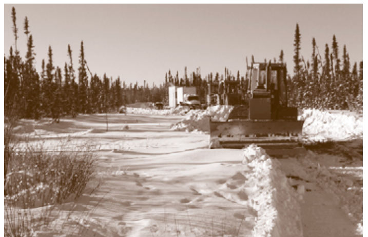
A winter road construction crew inches toward Tadoule Lake.
