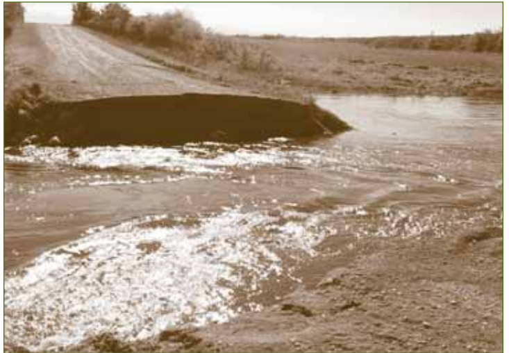
Heavy runoff can wash out roads and cut off emergency access for remote communities.
