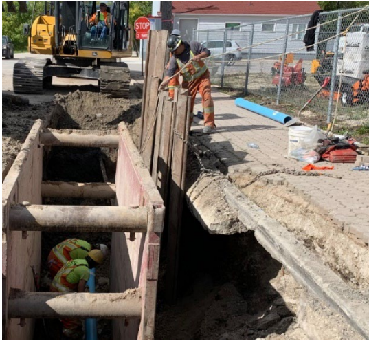
Town of Arborg Water Renewals
