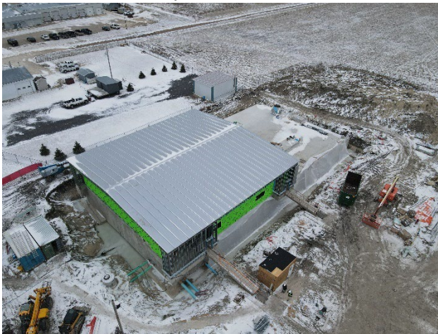
Town of Beausejour Water Treatment Plant
