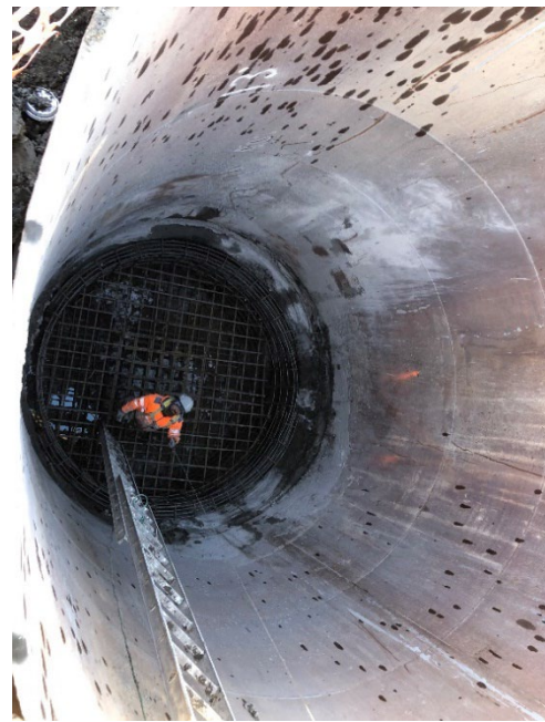
City of Morden Sewage Lift Station Upgrade
