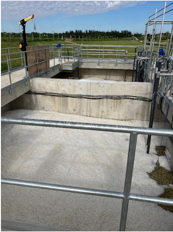
Town of Neepawa WWTF Phase 2 Upgrades
