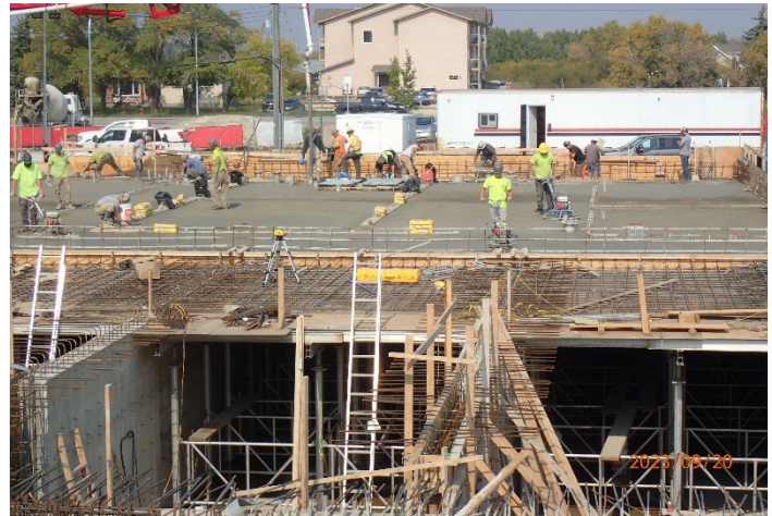
Town of Beausejour Water Treatment Plant
