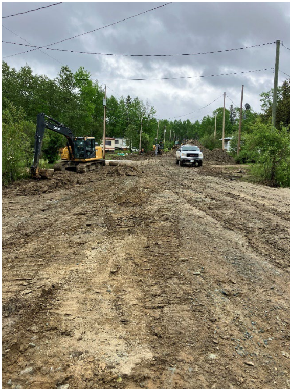
Community of Bissett Civil Works
