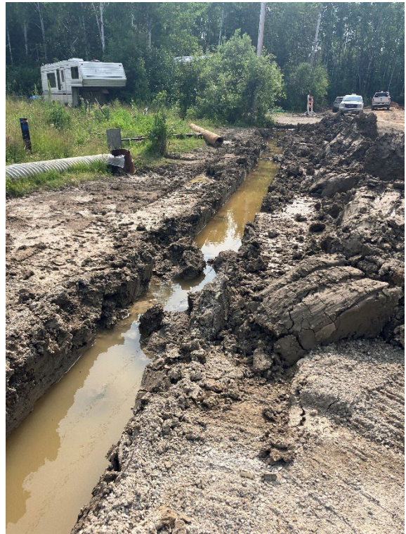
Community of Bissett Civil Works
