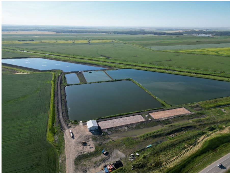
Town of Ste. Anne Wastewater Treatment Lagoon
