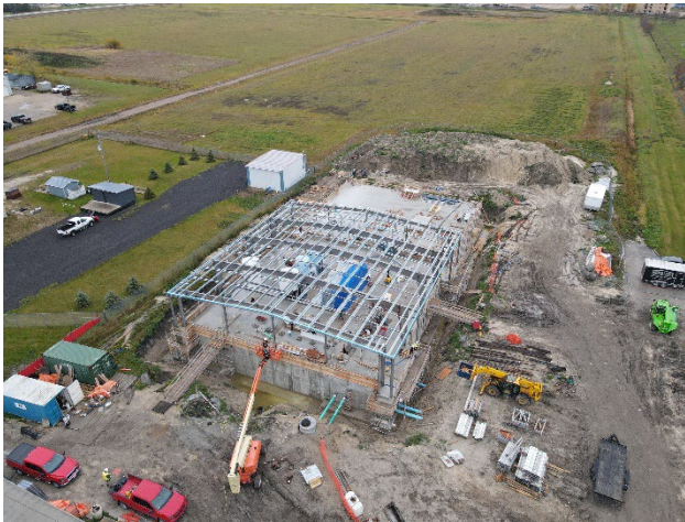
Town of Beausejour Water Treatment Plant
