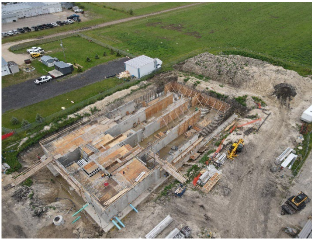
Town of Beausejour Water Treatment Plant
