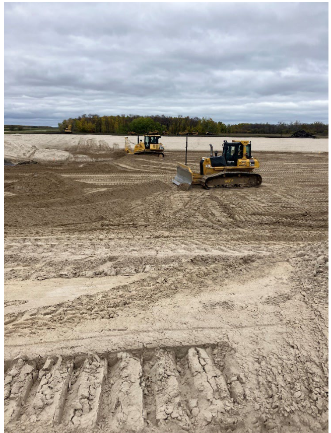
R.M. of St. Andrews Petersfield Wastewater Treatment Lagoon
