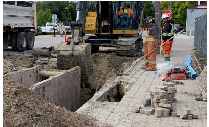
Town of Arborg Water Renewals
