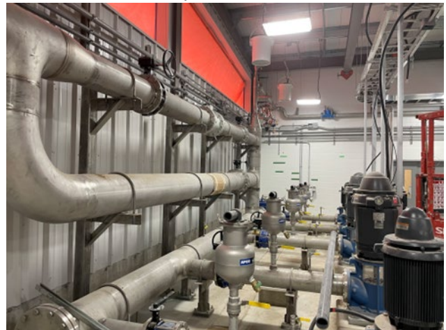
Town of Beausejour Water Treatment Plant
