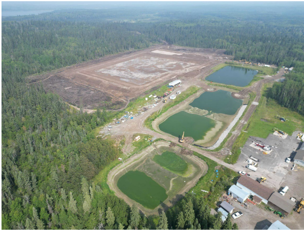
Paint Lake Provincial Park Wastewater Treatment Lagoon
