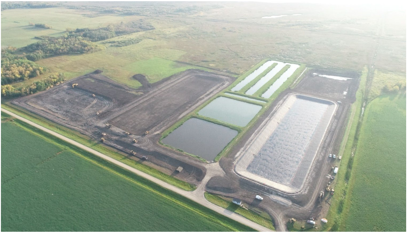
R.M. of St. Andrews Petersfield Wastewater Treatment Lagoon
