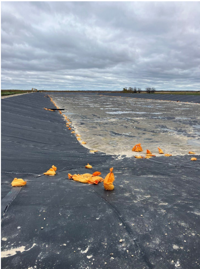
R.M. of St. Andrews Petersfield Wastewater Treatment Lagoon
