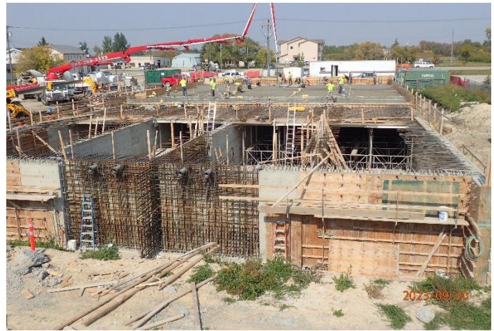
Town of Beausejour Water Treatment Plant
