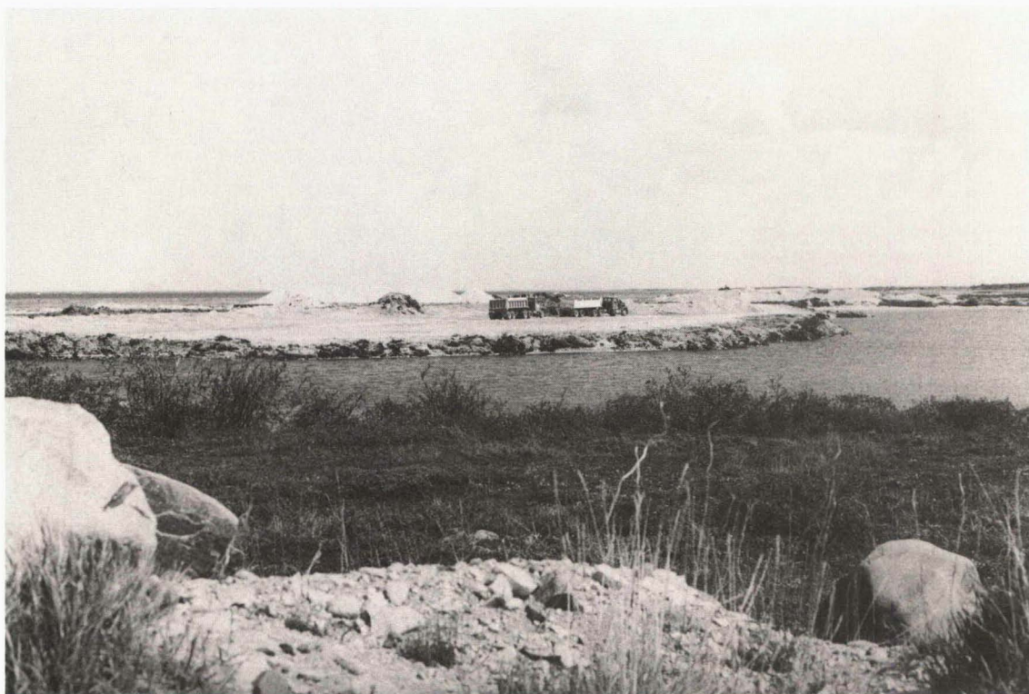
FIGURE 14. Sand and gravel removal from deposit 32034. Hudson Bay in background. Economic thickness of deposit and depth to water table is 1.0 m.
