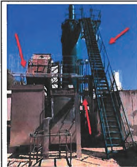
Stairways to stack platform
