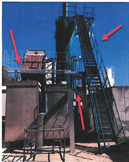
Stairways to stack platform
