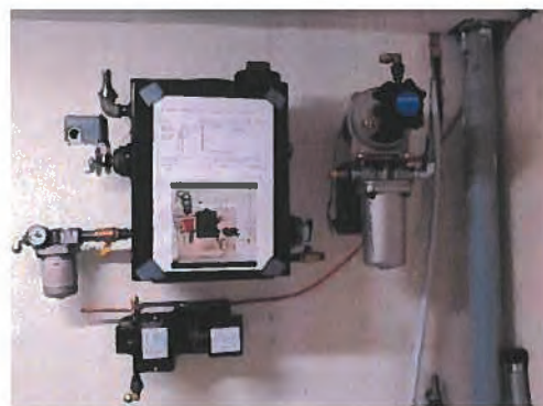
Oil Burning Unit Installation in Bunibonibee (Photo Tommy Weenusk)
