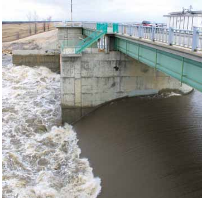
Floodway inlet control structure south of Winnipeg
