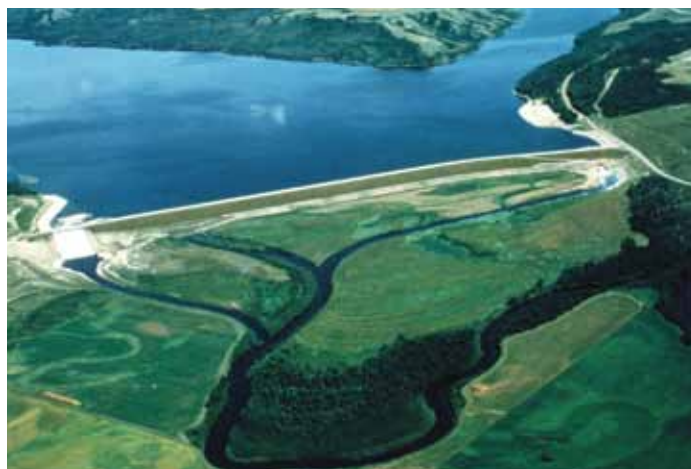
Shellmouth Dam structure and reservoir (Lake of the Prairies)
