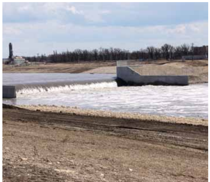
Floodway outlet structure north of Winnipeg
